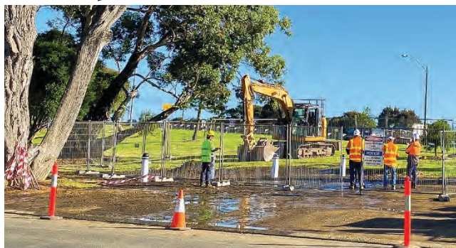
Work was underway in San Remo last week to repair a leak in the steel water main that supplies Phillip Island with water from Candowie Reservoir.
