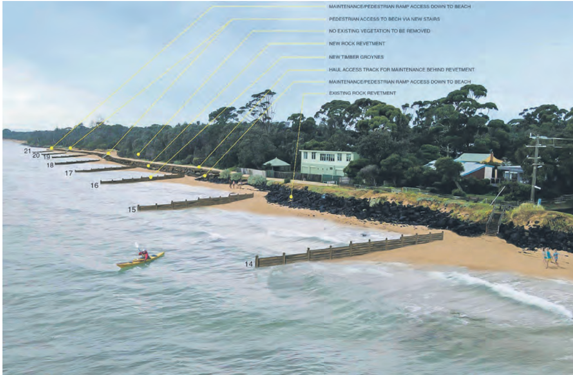
This artist’s impression shows the finished project with eight new groynes and the completed rockwall, with a pathway at the rear. The rockwall will be built after summer from February 2022.
