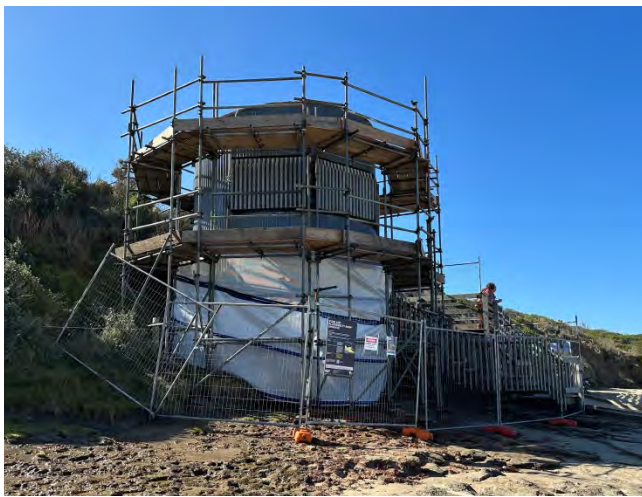
Work begun last week to repair the Smiths Beach Rescue Base, including repairing the corroded steel on the rescue base structure. It's due to be completed by mid-September.
