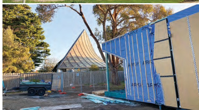
The building was constructed off site, then transported by truck to Cowes, with modules lowered into place by an enormous crane. Residents watched the transport and assembly with interest and can now inspect the completed building at the Open Day on February 11.
