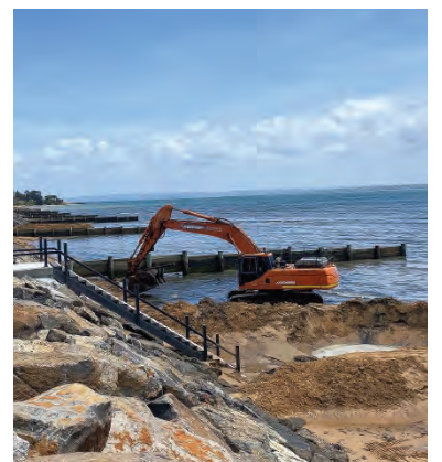
Cowes east’s $3.35 million, 360-metre wall metre boulder rock wall.
