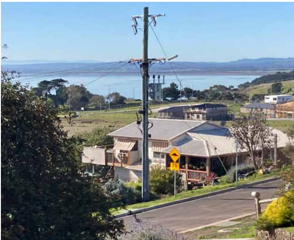
Power poles in Bonwick Street San Remo were removed last week, and three metre higher replacements (pictured) were installed. High voltage wires will be hung in three weeks time at the upper level, to service the new Westernport Views Estate.
