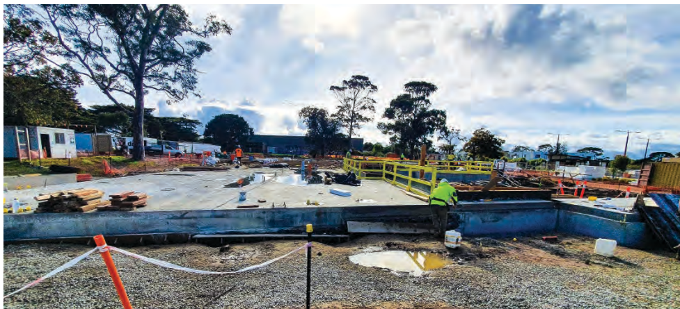
Construction crews have taken advantage of the break in the rain, with the entire concrete slab in the theatre area (stage 1) now poured.
