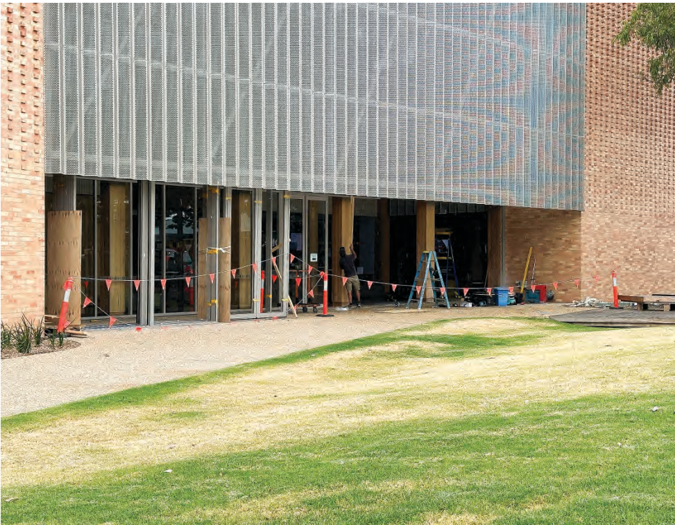
Last week, workmen were installing new passiv haus standard doors and windows from Germany at Berninneit, the new cultural centre in Cowes.
