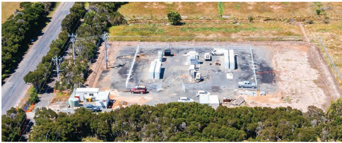
The $12 million, 10MWh lithium iron phosphate battery energy system on Gap Road will be officially launched on June 3, which will help replace diesel generation to power the Grand Prix. Photo courtesy of Mondo.
