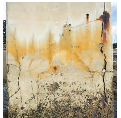
In recent years there were reports by the community of 'spalling' – where fragments of concrete break off a larger body and several cracks are visible in each pylon accessible by land at low tide. One crack over a metre-and-a-half long nears the width of a 50c piece in parts, with a small midden of shells nestled in its crevice.
