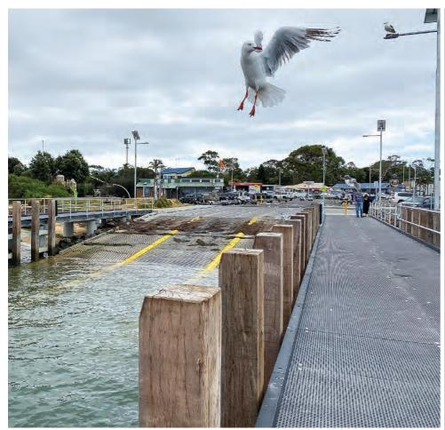
Following last year's \$4.5 million upgrade of the Rhyll ramp, the shire has received a grant to scabble the ramp, to provide more grip on the dangerously slippery concrete surface.
