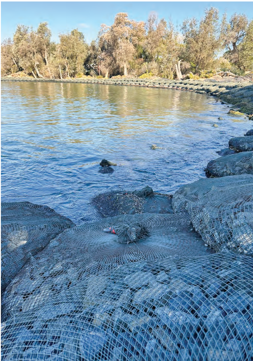
The new rock bag wall in Silverleaves' erosion hotspot came just in time for the biggest king tide of the season last Thursday.
