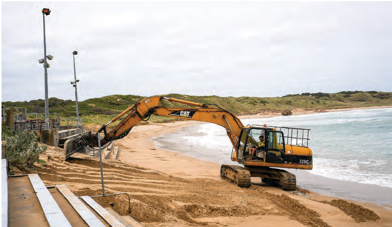
The Nature Parks is undertaking the beach nourishment at Summerland Beach, which involves adding large quantities of sand to counter erosion due to the impact of rising sea levels and storm surges.
