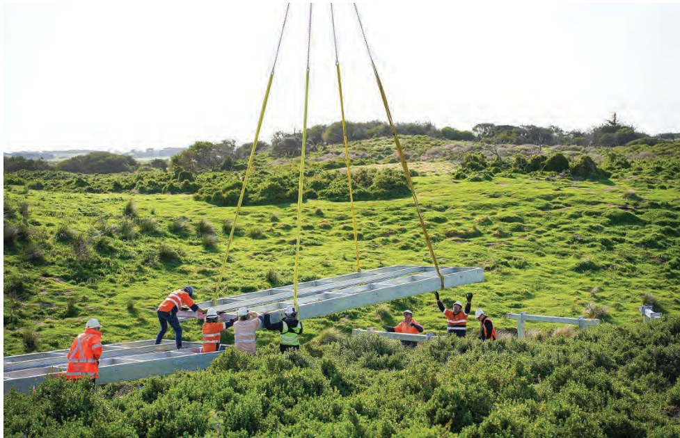
Workers were on hand to install the steel framework which was helicoptered in as part of the new boardwalk construction at the Penguin Parade.
