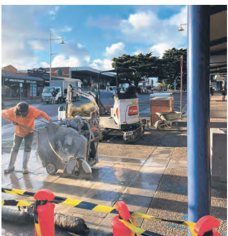
The concrete was removed to allow the existing wiring to be altered so new LED lighting can be installed.
