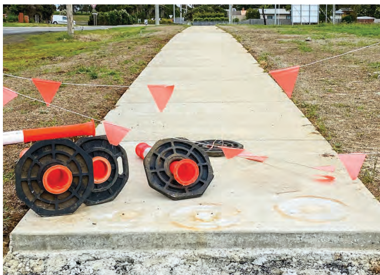
A newly installed footpath link ends abruptly with a 150mm drop. Footpath closed signage and witches hats designed to warn pedestrians have been displaced.
