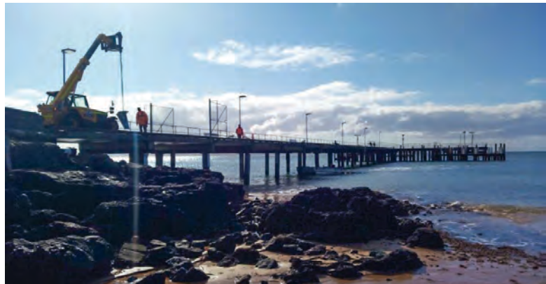
A new handrail is being installed on the eastern side of the pier and the walkway will be upgraded with new asphalt.
