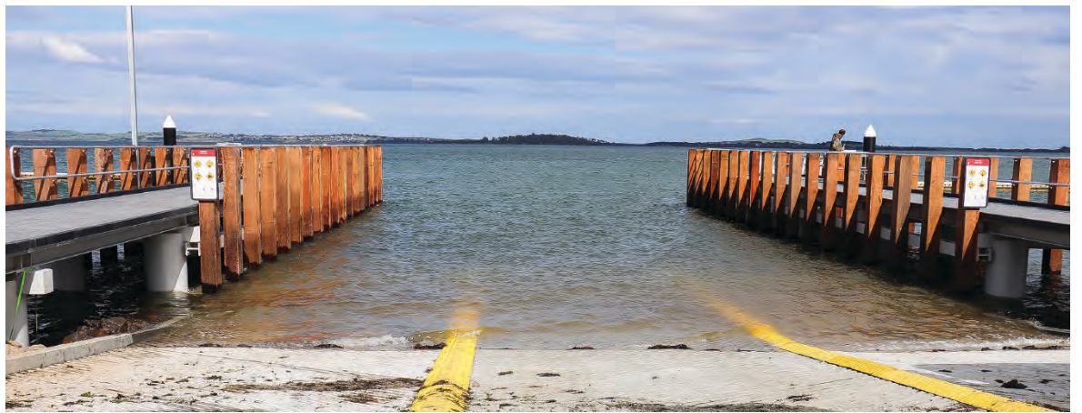
The $4.5 million redevelopment includes the replacement of the existing three-lane boat ramp with new concrete panels and extension of the lanes deeper into the water – enabling all-tide access.
