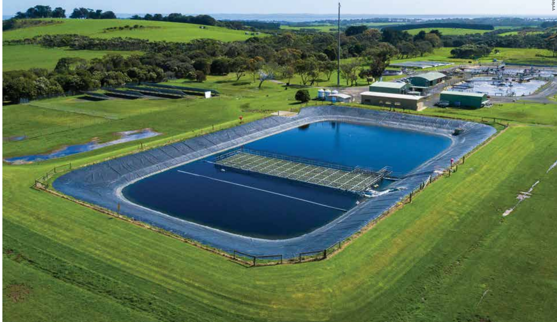
The floating wetlands system installed on a wastewater lagoon at Cowes Wastewater Treatment Plant.
