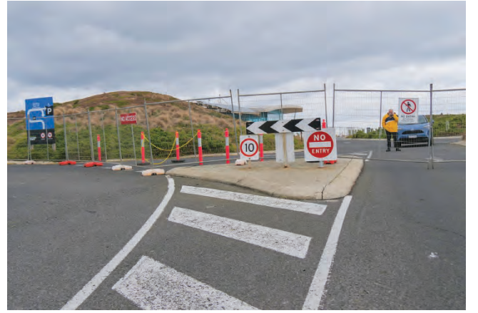
Phillip Island Nature Parks has advised the Nobbies precinct on the Summerland Peninsula has again been closed to visitors while further safety works are carried out, after strong winds earlier this month caused damage to the building's roof and solar panels.
